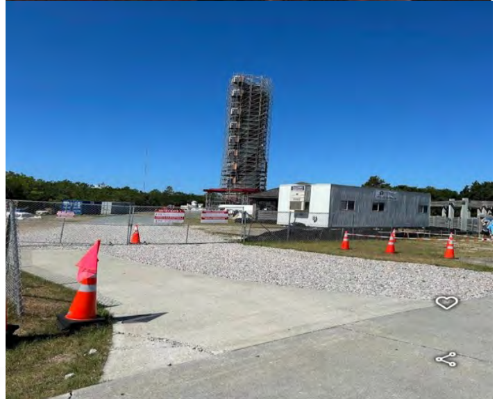
The Lighthouse at its relocated position about 880 metres further inland and now hopefully out of harm's way for the next decades. (The scaffolding is still in place to complete minor refurbishment)
