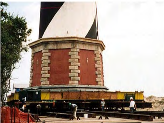
Preparation for another few millimetres of movement. Now you know why it took 23 days to relocate everything.
