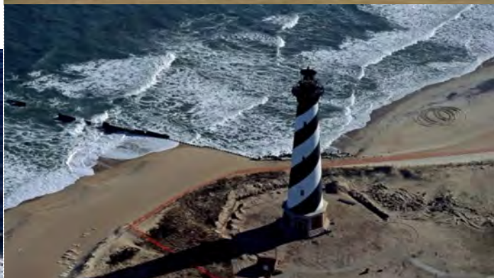
Showing the revetments on the sea side, a temporary solution
