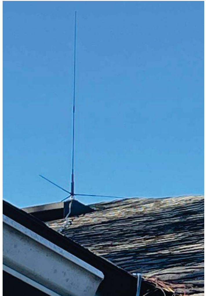
Figure 1. A stealth magnetic-mount mobile antenna on a metal roof vent with caulk around the mount for extra strength.
