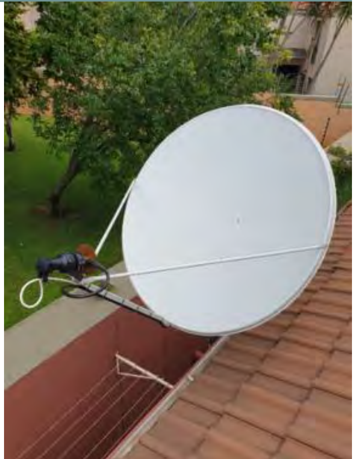
Figure 2. QO-100 dish Installation
