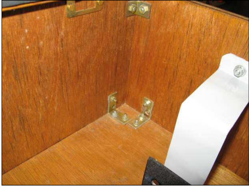
Close up of panel attachment brackets.
