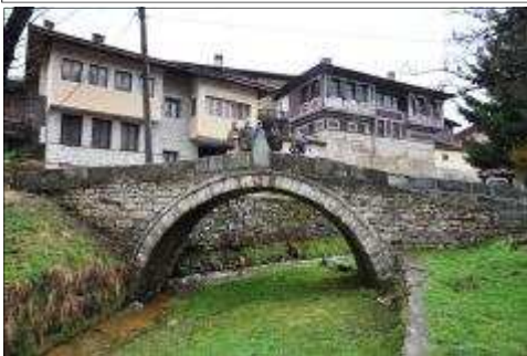
The bridge where the first shot of the April Uprising against the Ottomans was fired.
